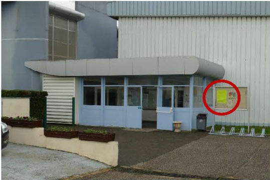
Gymnase, rue Charles Péguy
